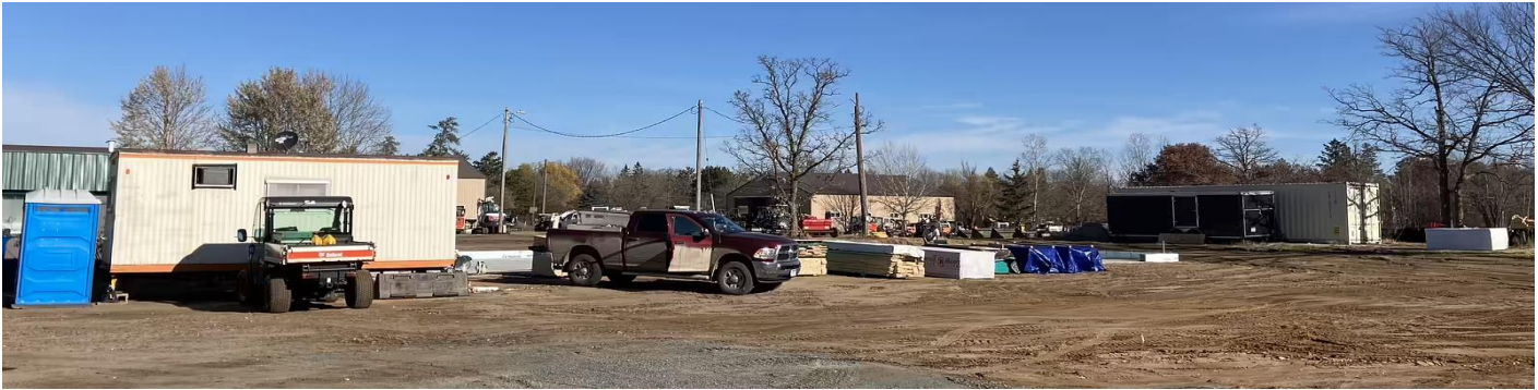
Hanson Contracting Shop, Irvine Ave NW, as of 11/1/2022
